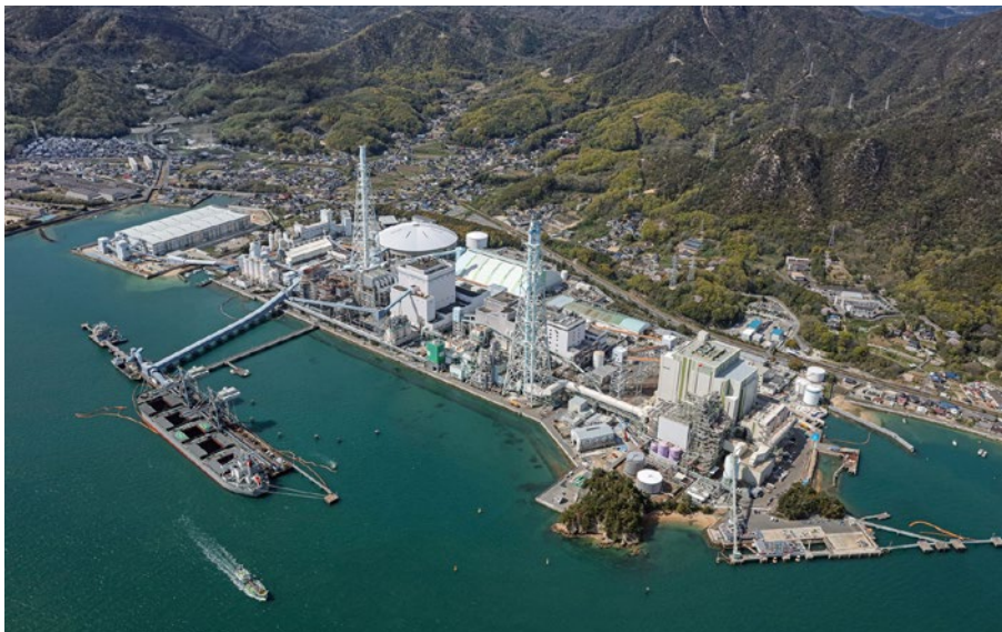
Takehara Power Plant (J-POWER)
