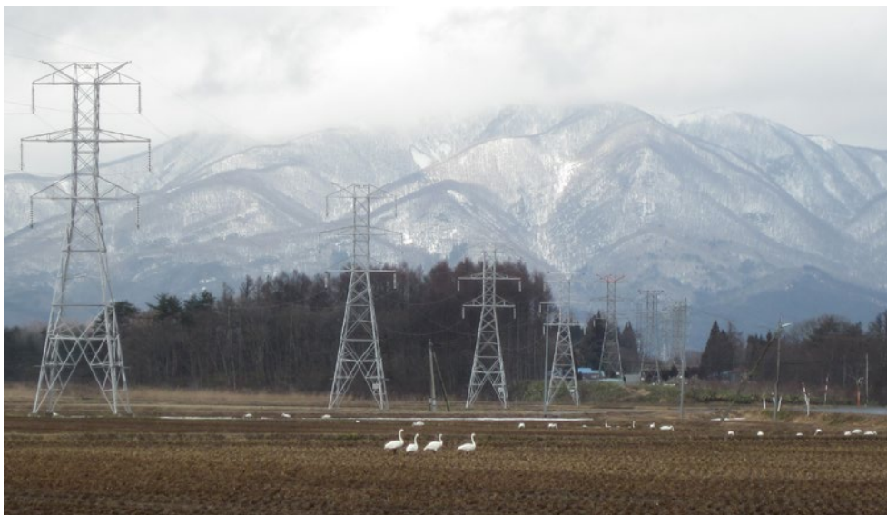
154kV Inawashiro Kyu-kansen transmission line (TEPCO Power Grid) Constructed in 1914 with the third longest (225 km) transmission line in the world at that time. Still in commercial use more than a century later. The transmission towers were manufactured by American Bridge.
