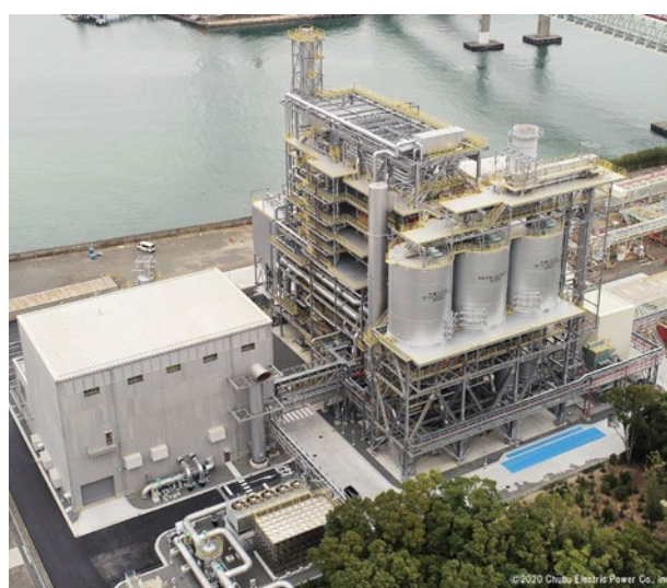
Yokkaichi Biomass Power Plant (Chubu Electric Power Co.) The Yokkaichi Biomass Power Plant is a woody biomass-fired power plant with an output of 49MW. Commercial operation started in May, 2020
