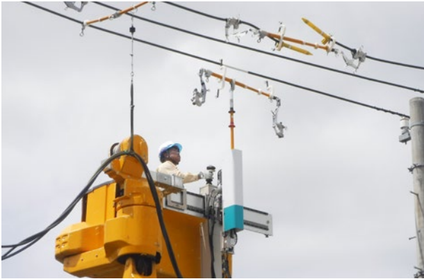
Assist Arms (Hokuriku Electric Power T&D)
