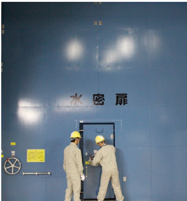
Entrance door and equipment hatch of Tokai II Power Station (The Japan Atomic Power Co.) made watertight Tokai II Power Station entered operation in November 28, 1978
