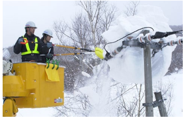
Removing snow from power lines (Hokkaido Electric Power Network)
