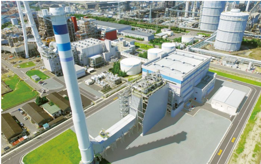
Unit 2 of Sakaide Power Station (Shikoku Electric Power Co.) Reentered service after conversion from oil to LNG-CC in August 2016.
