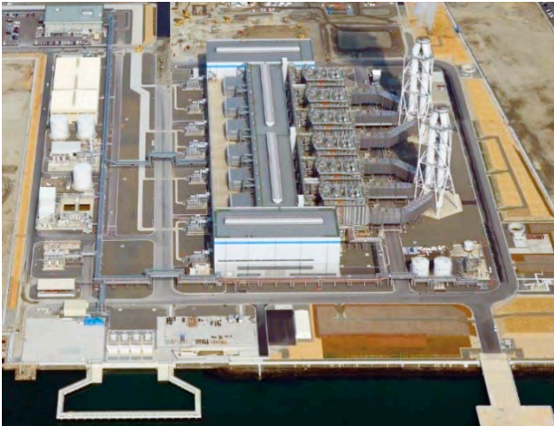
Nishi-Nagoya Thermal Power Station (Chubu EPCo)
