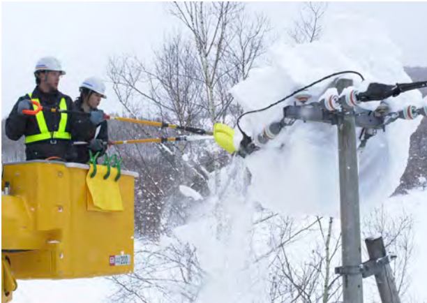
Removing snow from power lines (Hokkaido EPCo)
