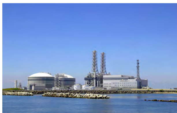
Shin-Sendai Thermal Power Station (Tohoku EPCO)
