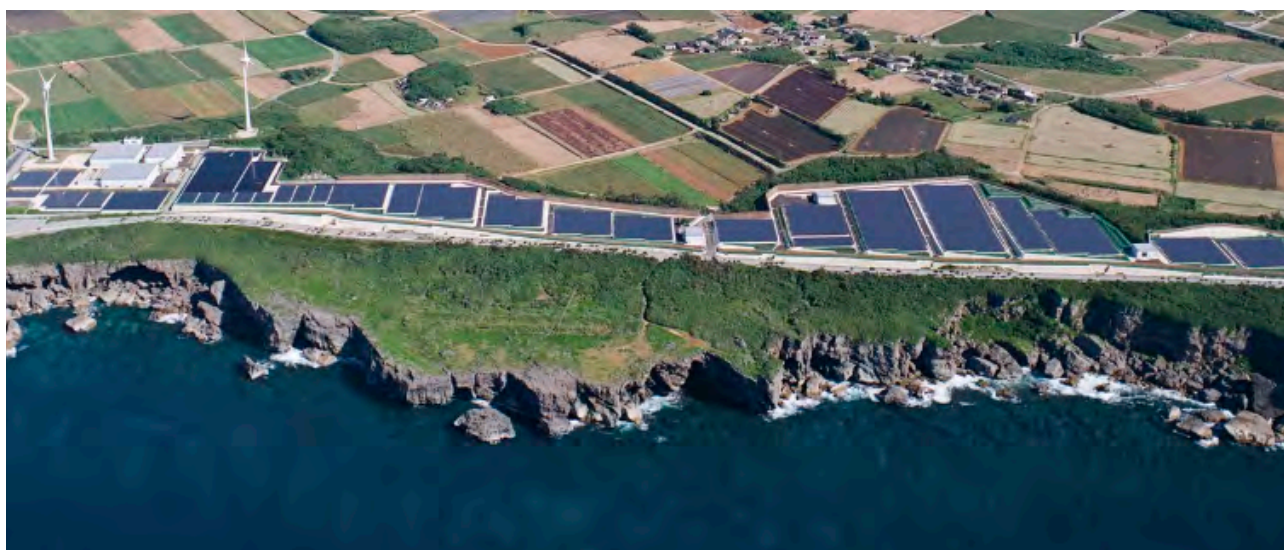
Utility-scale solar power generation testing plant (Okinawa EPCo)
