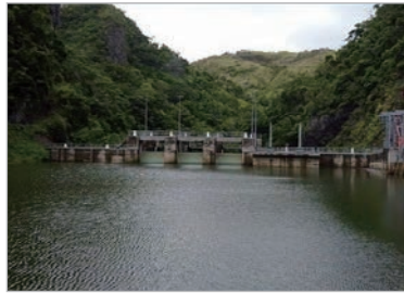
Nadarivatu Hydro Power Station
