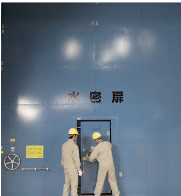
Entrance door and equipment hatch of Tokai II Power Station made watertight (The Japan Atomic Power Co.) Tokai II Power Station entered operation in November 28, 1978
