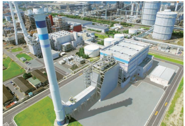
Unit 2 of Sakaide Power Station (Shikoku Electric Power Co.) Reentered service after conversion from oil to LNG-CC in August 2016.
