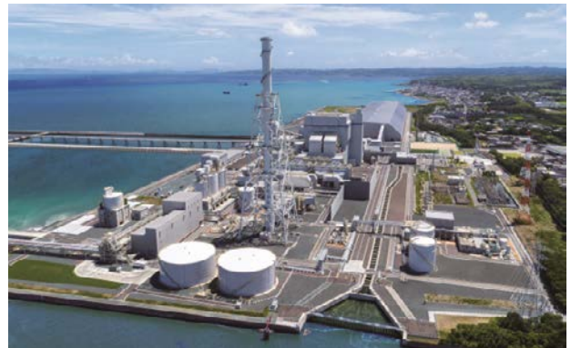
Taketoyo Thermal Power Station (JERA Co., Inc.) COD: August 2022* unit5 / Owner: JERA Taketoyo Thermal Power Station Unit 5 is a high-efficiency coal-fired power station that uses an ultra-supercritical (USC) power generation system, and it contributes to the stability of the electricity supply. By co-firing woody biomass fuel, it reduces CO 2 emissions as much as possible to mitigate environmental impact.
