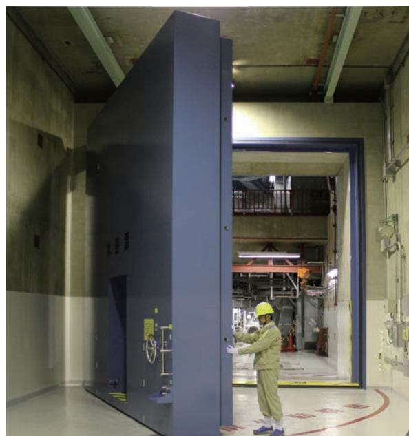
Entrance door and equipment hatch of Tokai II Power Station made watertight (The Japan Atomic Power Co.) Tokai II Power Station entered operation in November 28, 1978
