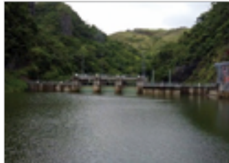
Nadarivatu Hydro Power Station
