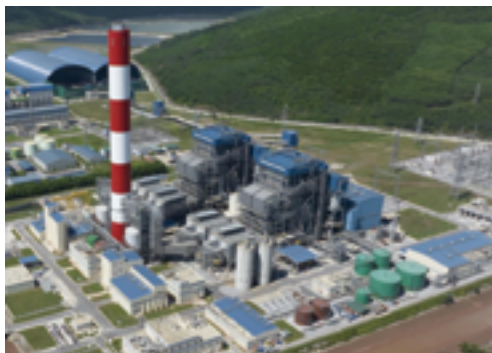
Power Plant Overview
