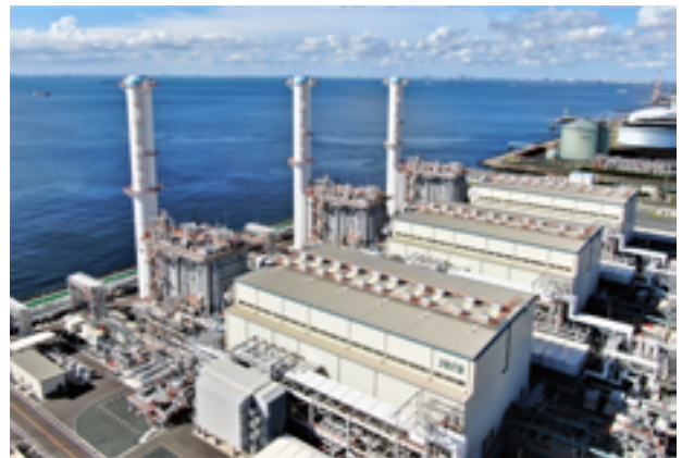
Anegasaki Thermal Power Station (New Units 1, 2, 3) (JERA Co., Inc.) COD: August 2023 (New Unit 3) / Owner: JERA Anegasaki Thermal Power Station (New Units 1, 2, 3) is a LNG-fired power station that utilizes a gas turbine combined-cycle power generation system (GTCC). The generating capacity is approximately 650 MW per unit (1,950 total) and will contribute to stable electricity supply. As a world-leading high efficiency power station, it mitigates environmental impact by reducing CO2 emissions.
