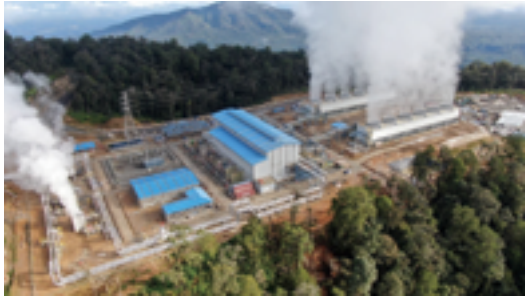
Power Plant Overview
