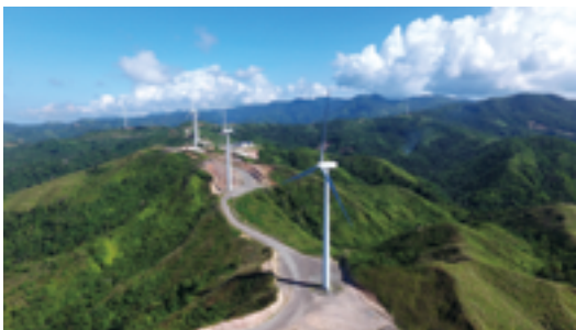
Nabas Wind Power Plant, owned by PetroGreen Energy Corporation
