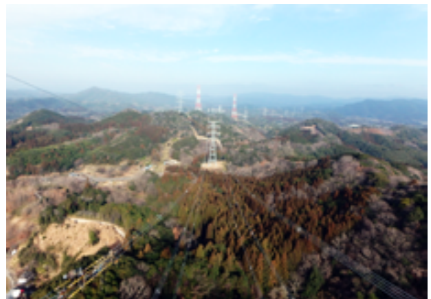
The 500,000-V Hyuga Trunk Line (Kyushu Electric Power Transmission and Distribution) Construction: June 2022 / Operators: Kyushu Electric Power Transmission and Distribution Co., Inc. Special note: The 500,000-V Hyuga trunk line was constructed to build the 500,000-V loop system in the area between northern and southern Kyushu. The facility aims to prevent widespread power outages during planned updates to aging 500,000-V infrastructure.
