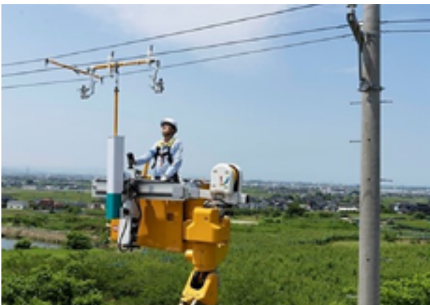
Assist Arms (Hokuriku Electric Power T&D) Hokuriku Electric Power T&D utilizes "Assist Arm" robots jointly developed with universities and manufacturers to aid power distribution workers. In the near future, these will reduce labor requirements and improve efficiency by automating some work.
